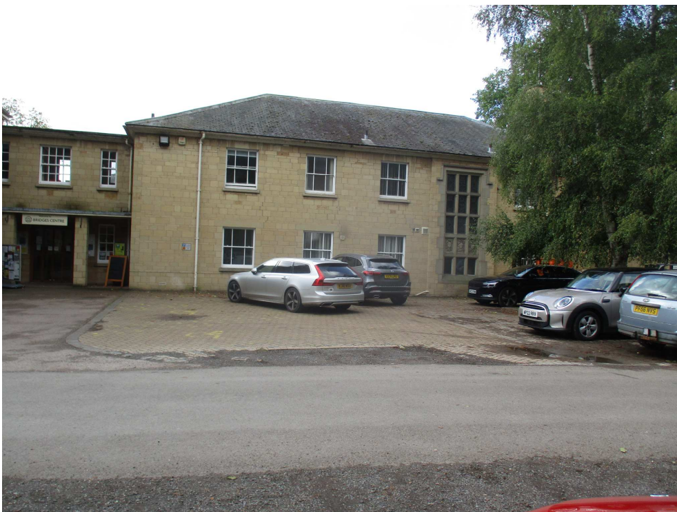
Photo 29 Some uneven surfacing to parking area.
