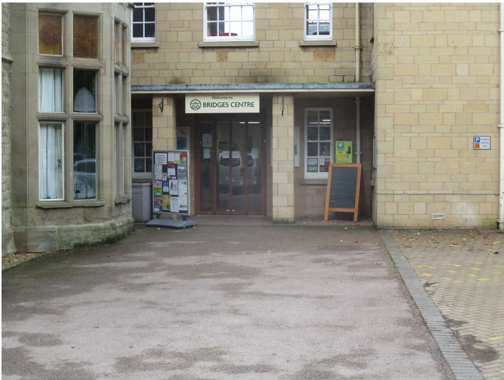
Photo 28 Level approach and auto entrance doors
