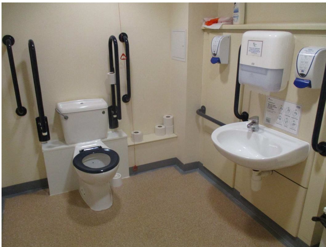
Photo 25 Peninsular layout accessible WC facility.
